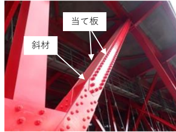
Fig.1 Application of reinforcement using cover plate
