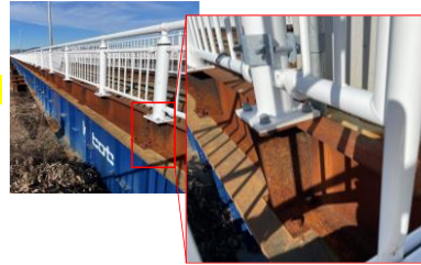
Fig.1 Guardrail post structures for temporary bridges (example)
