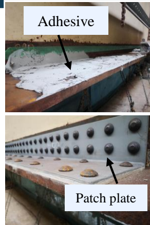
Fig1. Typical patch plate-repair
