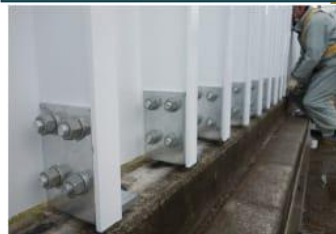
Fig. 1 GFRP wall rail joint
