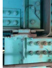
Fig. 2 Hinge bearing
