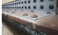
(c) High-strength bolted joints with adhesive
